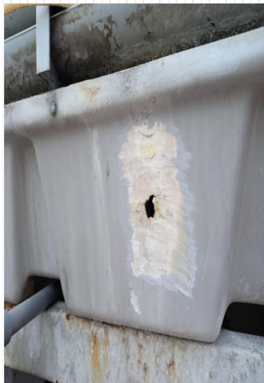
Cooling Tower FRP Leak Repair PT TD Automotive Compressor Indonesia
