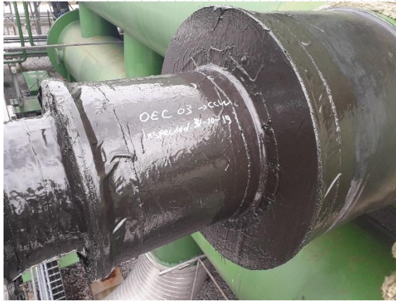
Pipe Thickness & Leak Repair SARULLA Ltd- Tarutung Medan
