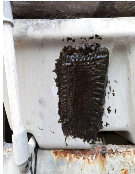
Cooling Tower FRP Leak Repair PT TD Automotive Compressor Indonesia
